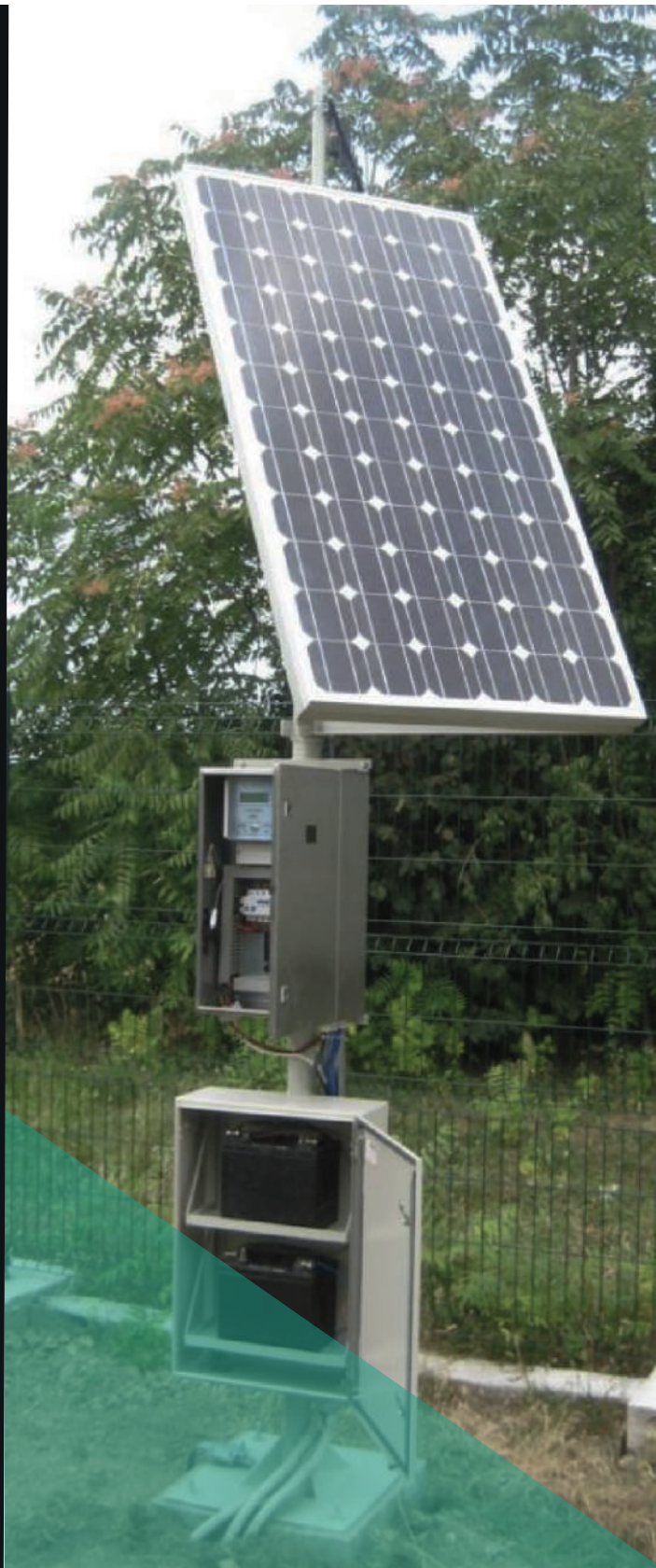
Solar powered installation and communication via GSM Dana network.
